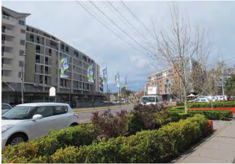
Contemporary multi-unit residential development
