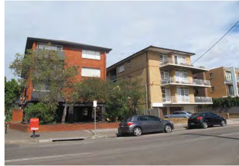
70's residential unit blocks
