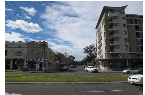
Complimentary old and new architecture
